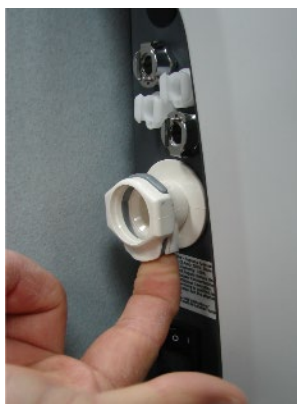
To disconnect, press gray button on the outlet. This will release and eject the air line.
