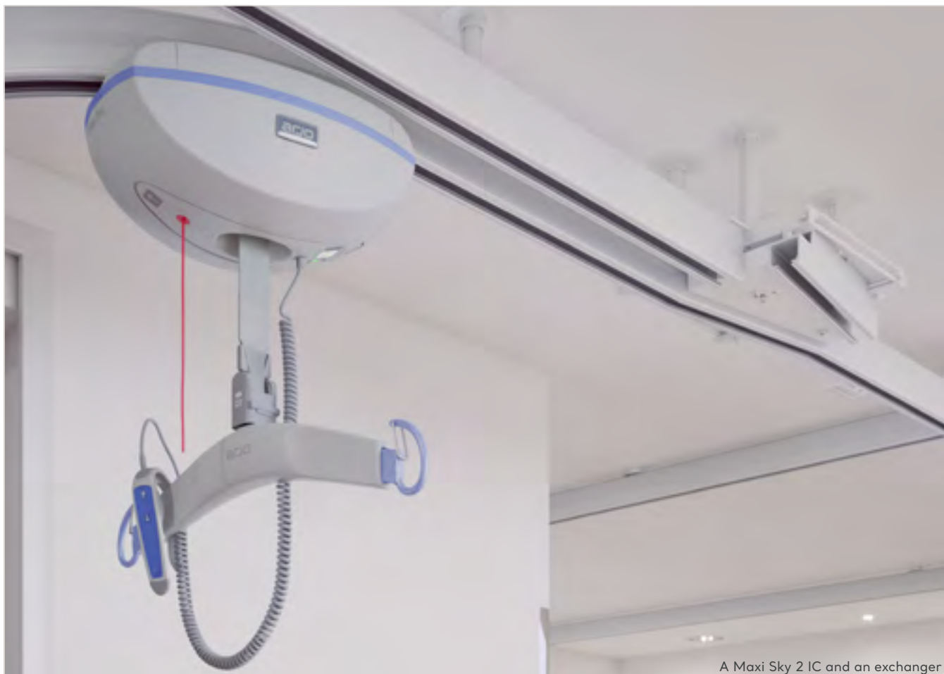
Maxi Sky 2 IC entering in an exchanger
